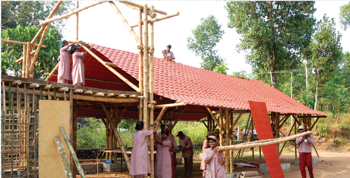
Construction Using Bamboo
