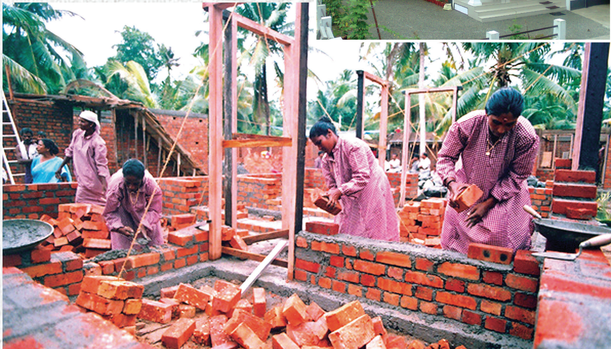
Re-construction - Tsunami - Alappad Panchayath
